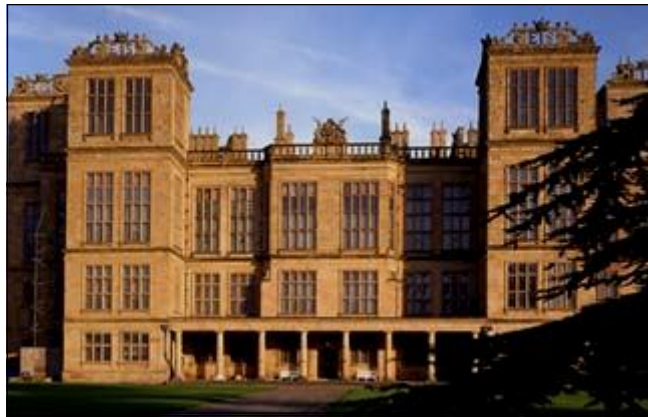
Hardwick Hall, Derbyshire. built in the 1590s
